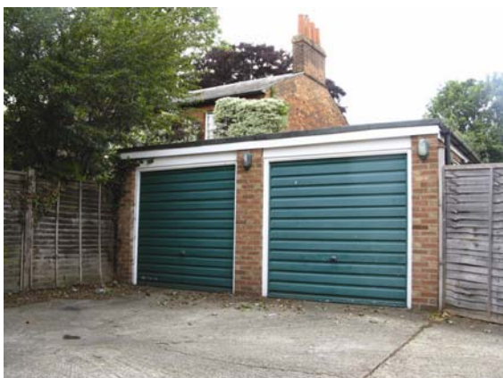
Garages at the back of No.4a Stevenage Road
