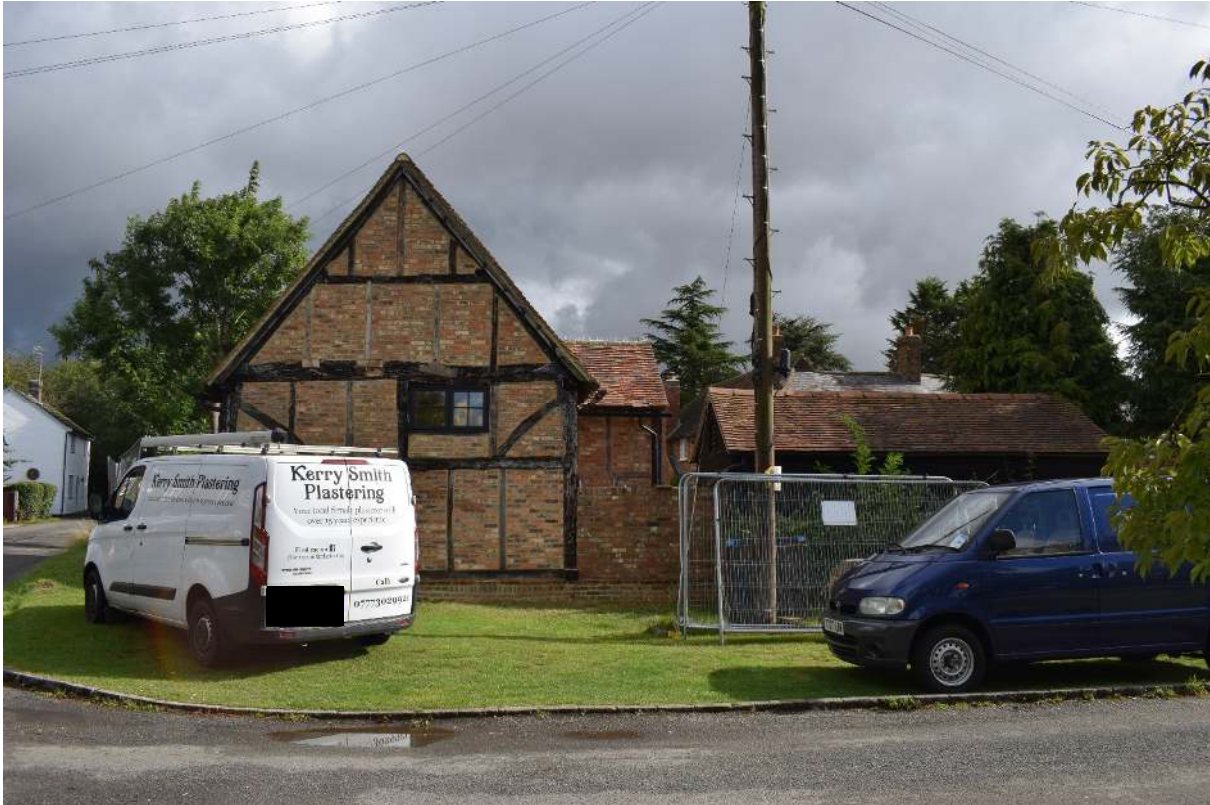
Figure 2.3 The Grade II listed Barn at Entrance to Green Farm on East Side of Green, looking northeast. This makes a positive contribution to the character of the Conservation Area. Along with planting, the barn obscures view of the Grade II listed Green Farm on East Side of Green.
