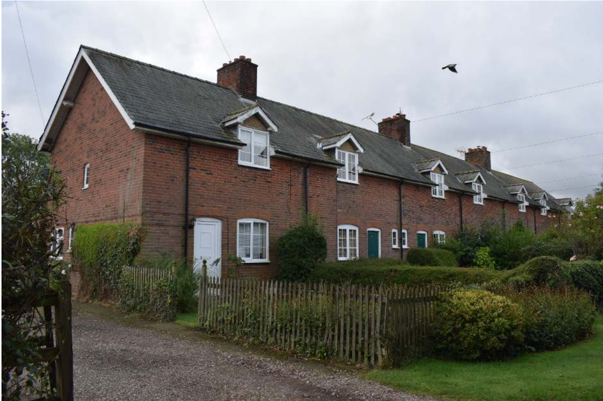
Figure 2.4 19 th century terrace on of the south side of the green, looking southwest. These are workers cottages orientated toward the green and representative of the linear form of historic buildings within the Conservation Area. The presence of steep gable ends overhung by deep eaves with barge boarding and prominent purlins is a feature of a number of buildings within the village.
